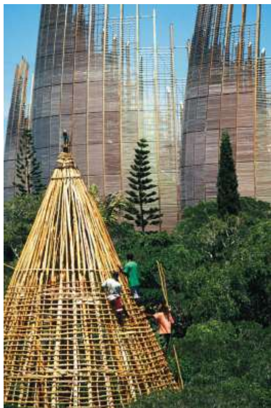
Fig. 4b. Renzo Piano's Jean-Marie Tjibaou Cultural Center, New Caledonia [b. Kanak roof construction within the site, bottom.]
