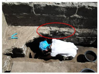
**Figure 28:** Encircled portion in the photo is the crumbling lime mortar foundation (Photo by Angelus Sales).
